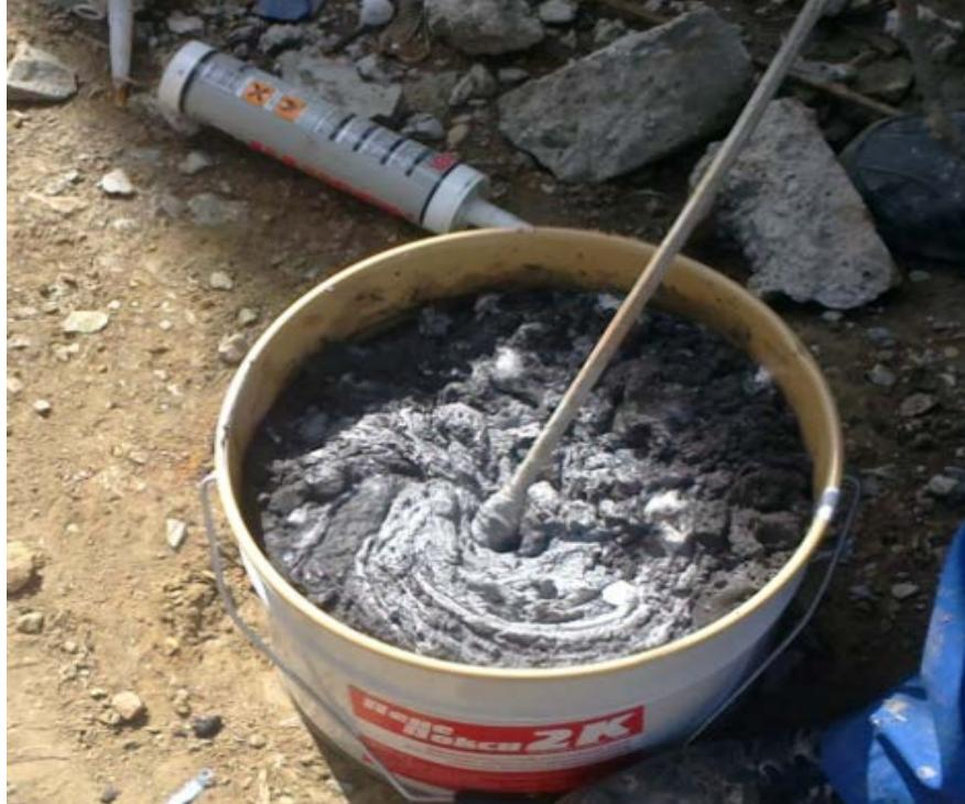
A photograph showing a white bucket with a red label containing grey adhesive. A power drill with a mixing attachment is inserted into the bucket, creating a swirling motion in the adhesive. In the background, a grey tube labeled 'ПеноПокси 2К' lies on the ground. |
